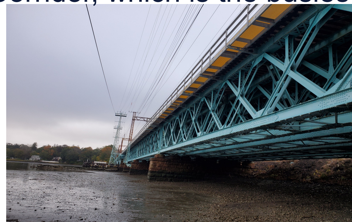
Figure 1: Cos Cob Bridge, Greenwich, CT (Built-in 1904; Span 3 length: 122'-10"; Height: 15'; Track 4 Width: 7'-6"; Total no. of Tracks: 1)
