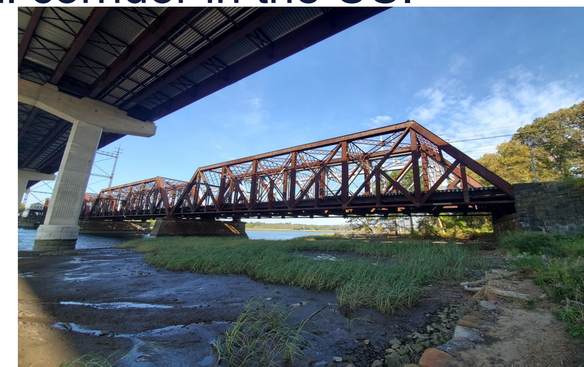
Figure 2: Devon Bridge, Stamford/Milford, CT (Built-in 1906; Span 7 length: 217'-7"; Height: 40'; Width: 30'-10"; Total no. of Tracks: 2)
