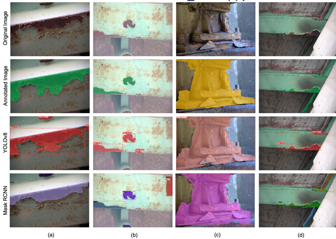
Figure 1, Original test images (first row), corresponding annotations (second row), prediction of YOLOv8 trained model (third row) and prediction of Mask RCNN trained model (forth row)
